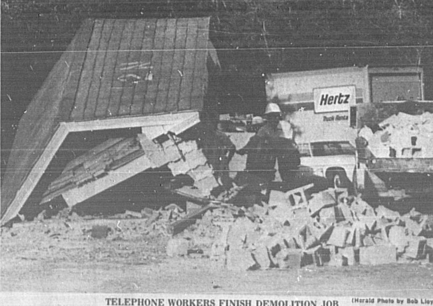
TELEPHONE WORKERS FINISH DEMOLITION JOB (Herald Photo by Bob Lloyd)
