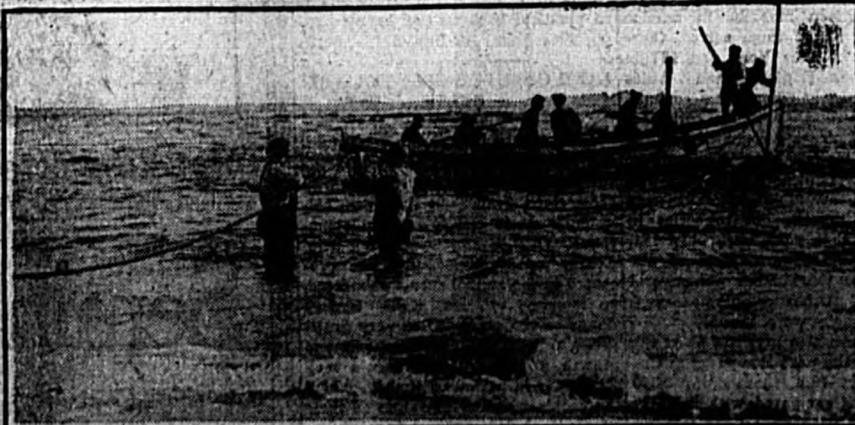
Here is the start of the laying of the eighteenth cable connecting the United States and Europe at Rockaway, N. Y. Despite the increasing use of radio, popularity of the cable still grows. The new one will be the longest and fastest.
