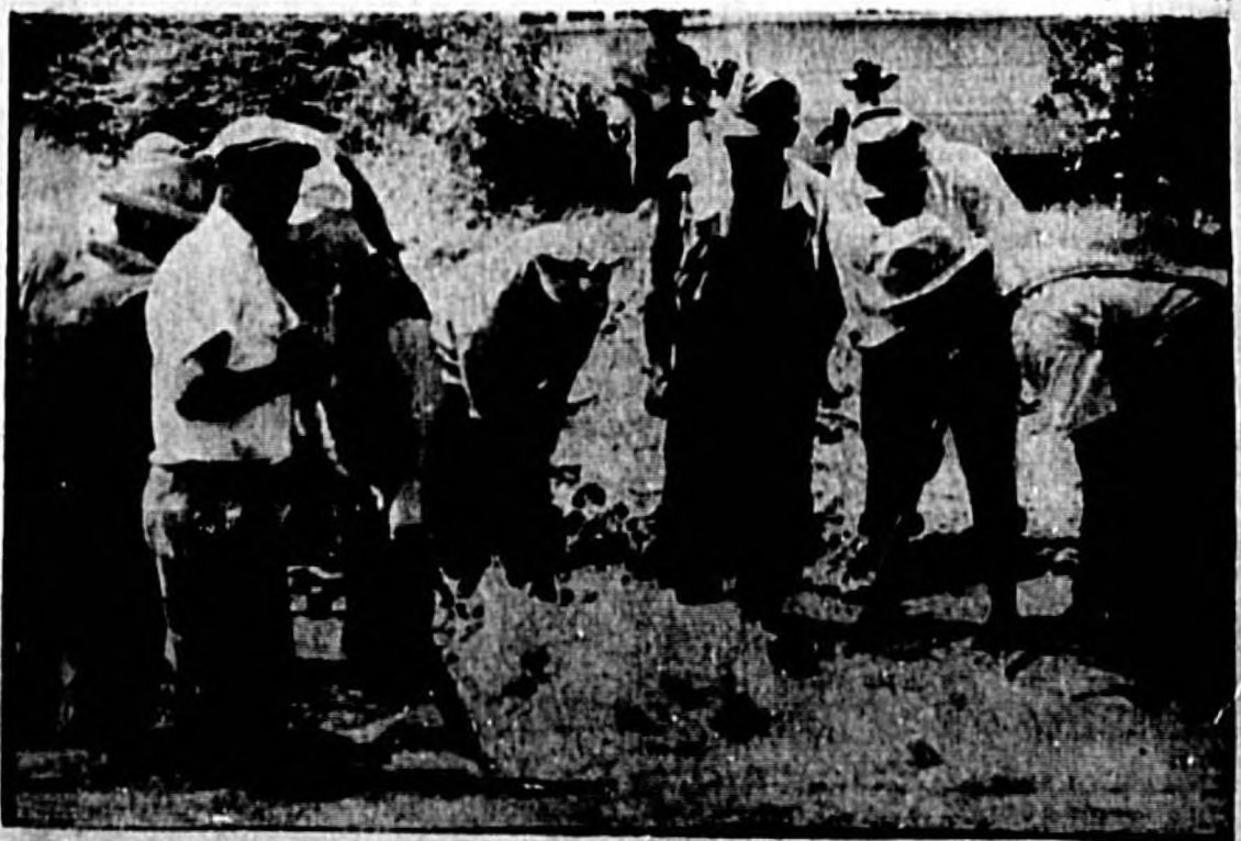
CITY CREWS PUT an eight-inch water main back into operation at First St. and French Ave. Sunday morning. Workmen are removing dirt and sand from around the pipe preparatory to the repair. (Staff Photo)
