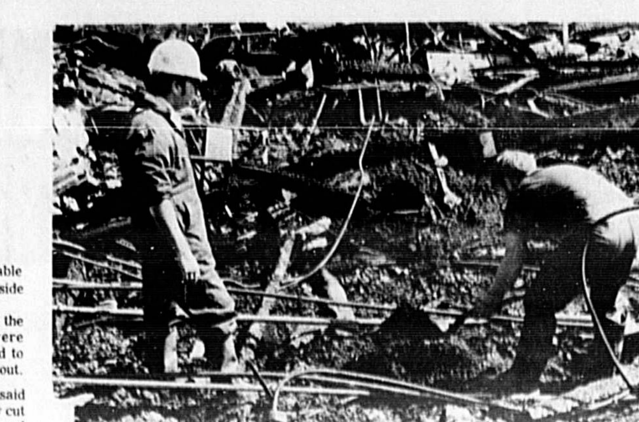
HAROLD DEESE (left) of the State Fire Marshal's office and Lt. Jim Dwoyer of the Sanford Fire Department sit through the ruins at Crooms High where fire destroyed most of a 46-year-old building last Thursday. Lt. Bill Lee of the Sanford Fire Department also assisted in the probe which is continuing. Sanford Fire Chief G. M. Harriett said some samples from the ruins have been sent to Ocala for analysis.
