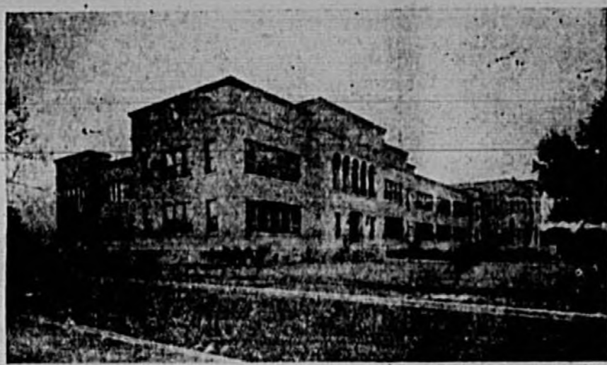
The Seminole County High School, constructed in 1925, is the pride and joy of many Sanford mothers and their children. The shade of the trees seen in the left foreground, is but a small part of a grove which was saved for posterity by the prompt action of the Garden Club at the time the school was built.
