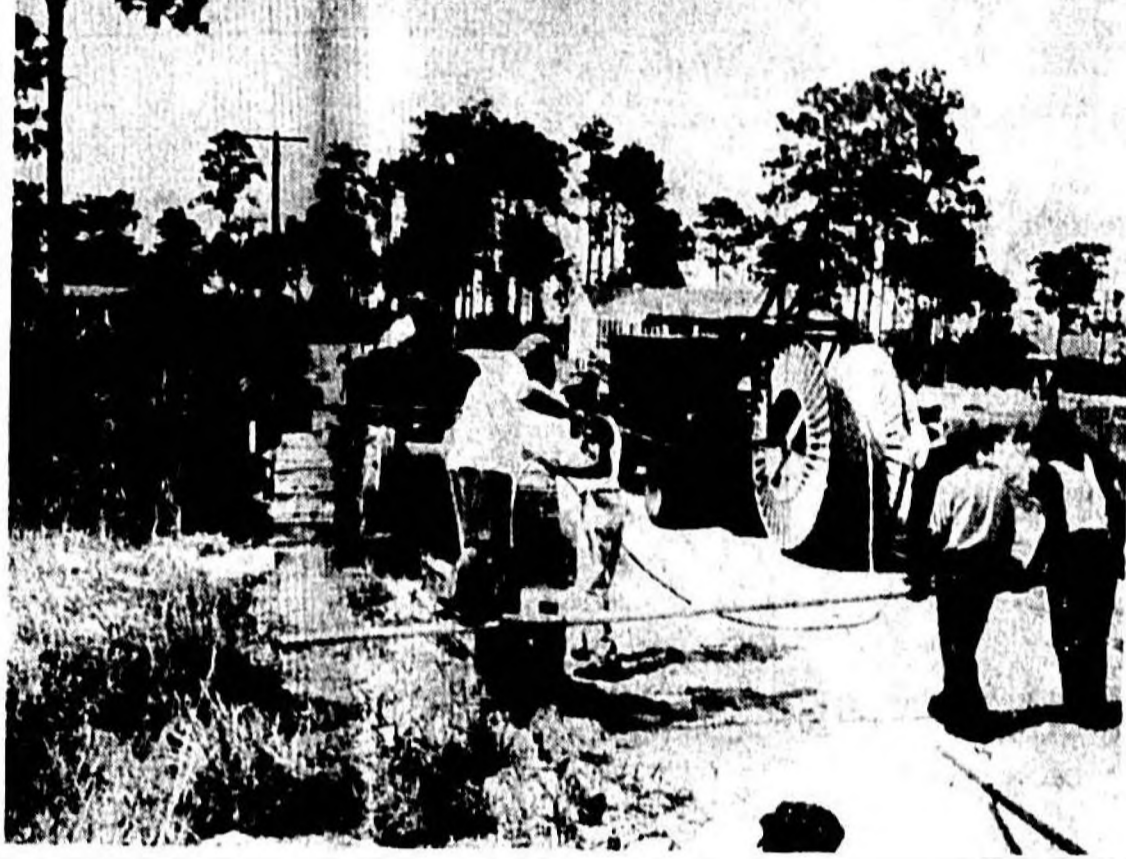
Workers of the Southern Bell Telephone and Telegraph Co. are shown laying telephone cable from Enterprise to the new community of DeBary and Plantation Estates. Following the completion of the connection with the local telephone exchange, the cable will be laid on the ground in a trench cut by the big digger at right and laid through a pipe on the approach to DeBary. Photo by Cox.
