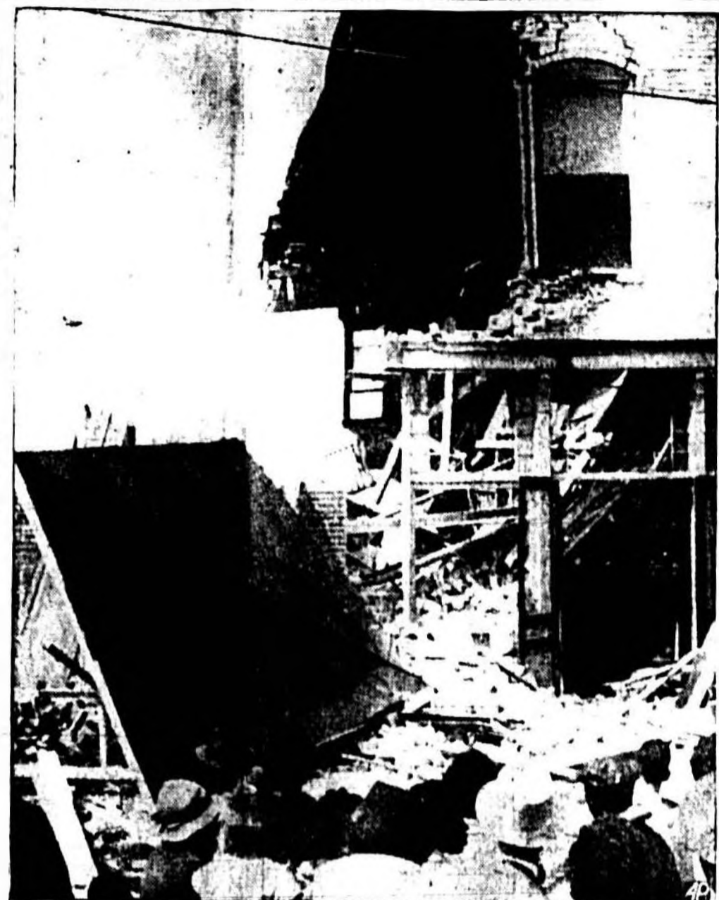
In this shambles, all that remains of a building that collapsed in the business section of the City, Ala. 11 men died and 26 others were injured, enough to require hospital treatment.
