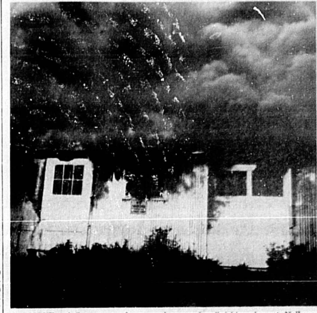
SMOKE and flames pour from warehouse and refinishing shop at Noil Furniture Company in Casselberry as sign warns in vain. "No Smoking" and "Keep fires away." (Herald Photo)
