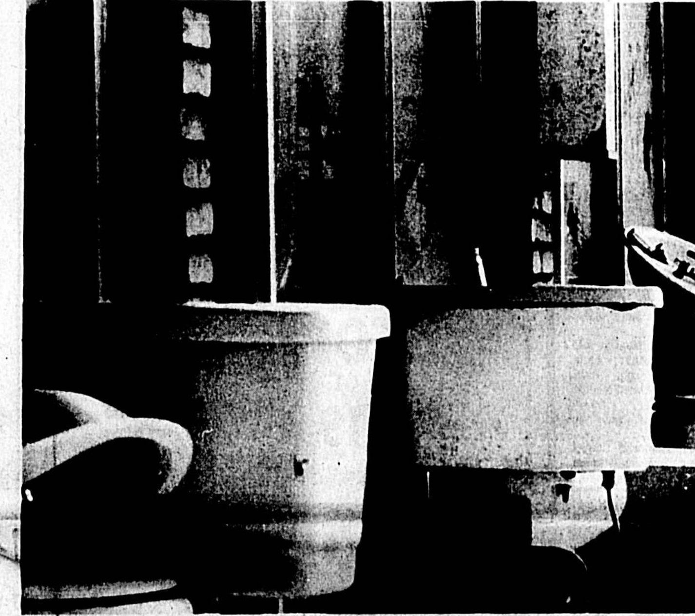
Outdoor Plumbing? No, they're not taking a giant step backwards for mankind by moving toilets outdoors. The commodes are awaiting installation at the Cavalier Motel on U.S. 17-92. Job foreman Joe Whitley ponders the view at the motel, which is scheduled to open in mid-January.
