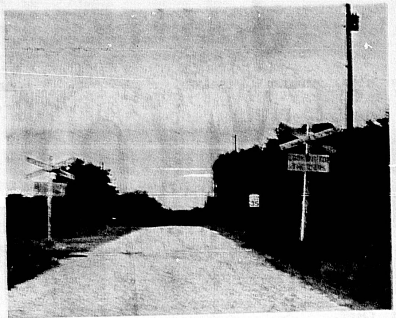
SR 427 crossing at Elder Springs.
