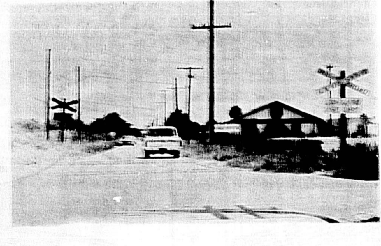
Grapeville Ave.-McCracken Rd. crossing.
