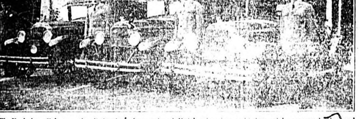
To Berkeley, Cal., goes the distinction of operating the first police fleet which is completely radio equipped. In line with his policy of providing every scientific aid for his men, Police Chief August Vollmer, well-known criminologist, sponsored installation of fixed-tuned short wave sets under the rear decks of these...
