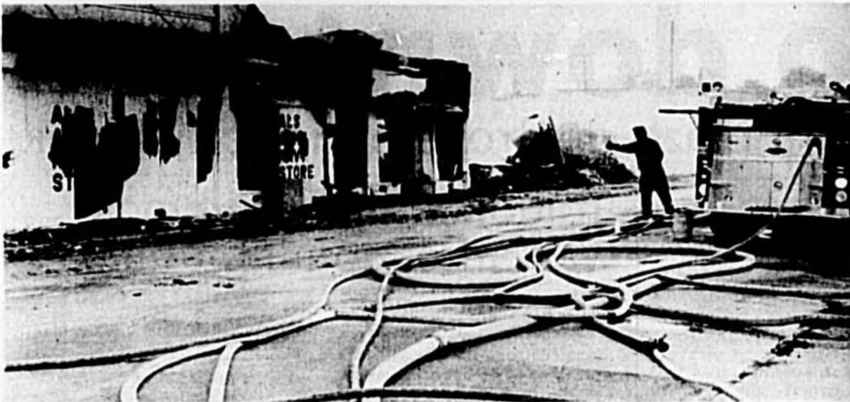
Firefighter John Smith throws debris off the roadway.
