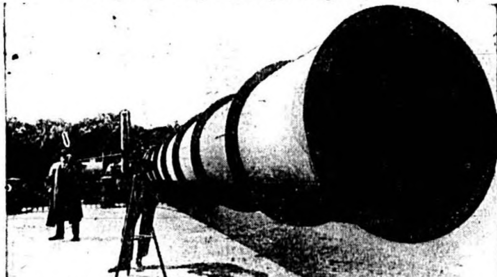
BERLIN—The gigantic Treppeauer Telescope here has seen service for the past 25 years. The telescope weighs 410 tons and is 70 feet long. With the necessary weights used in conjunction with the telescope, its total weight is 2,600 tons. The 25th anniversary of the Treppeauer Observatory is being celebrated this month.
