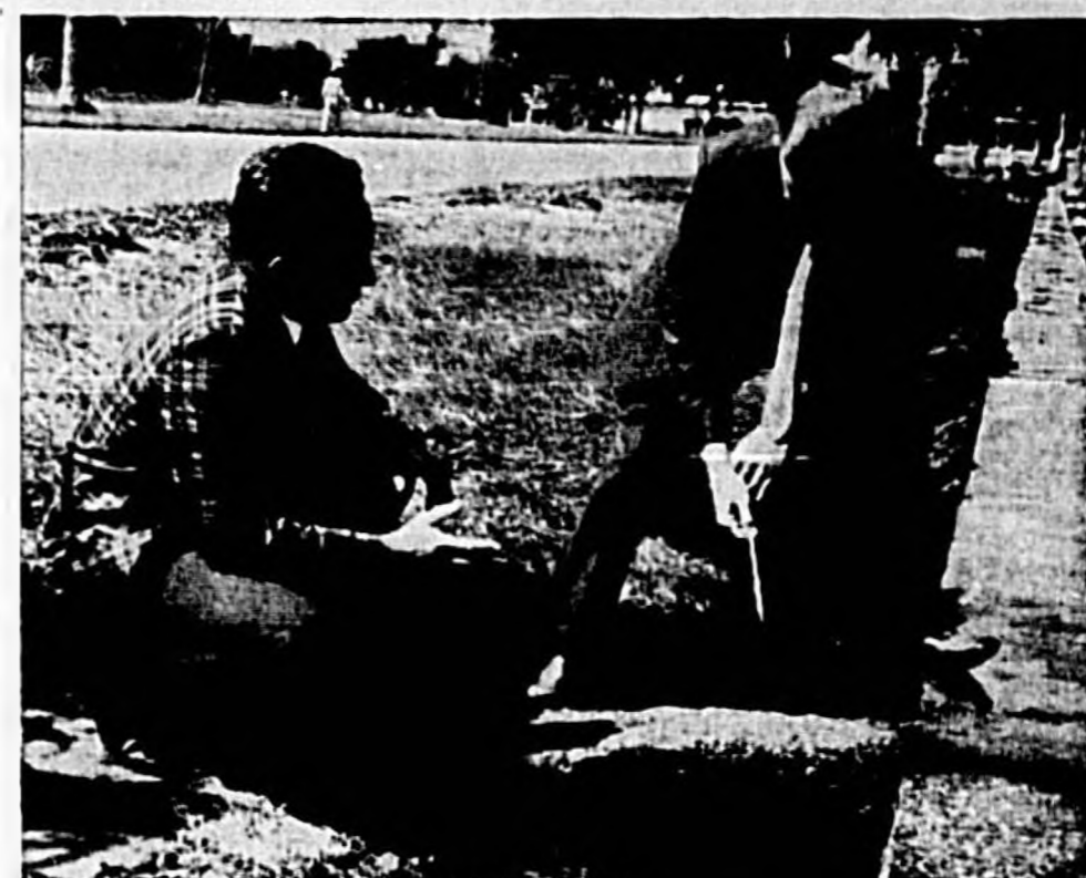
EXAMINATION OF THE SUPPORTS of the bulkhead along Sanford's waterfront was made convenient by recent Hurricane Dora which washed away some soil surrounding the supports. Here Reynolds Clark, planner with the Connell engineering firm retained by the city make a cursory check of the situation with City Manager W. E. Knowles. Clark is doing the preliminary planning work on the waterfront development plan.
