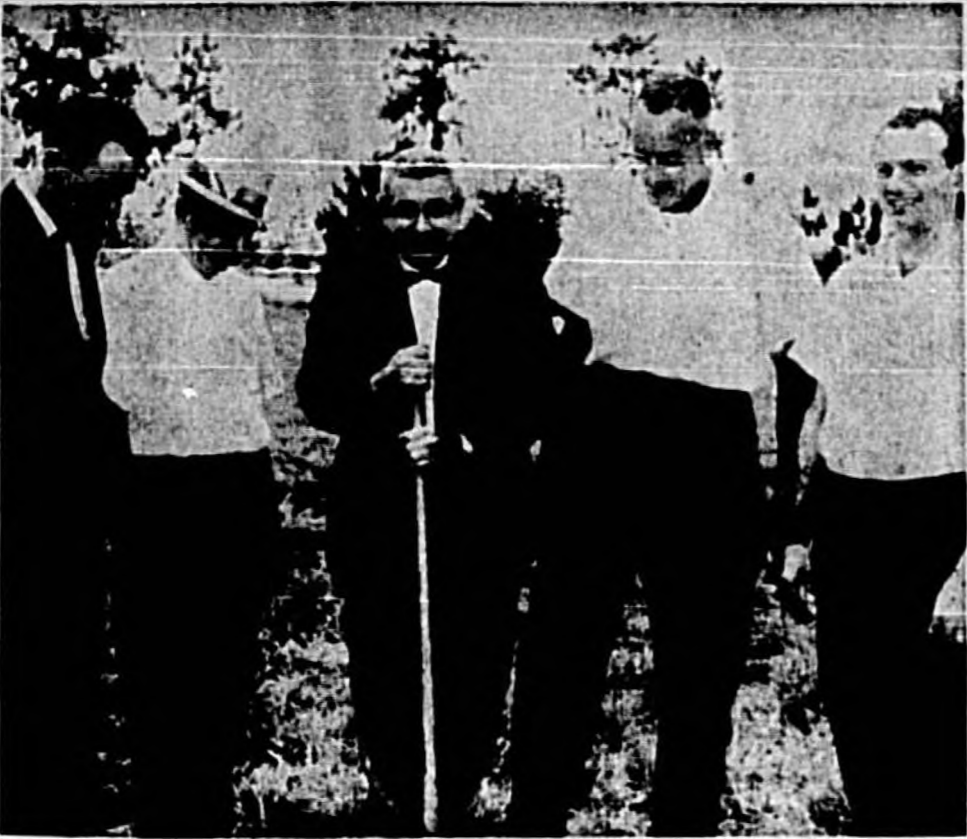
GROUND-BREAKING ceremonies for the new $400,000 Retirement Life nursing home on five acres off Highway 17-92 south of St. Ann's Church at DeBary were held Friday afternoon. Taking part in the picture, left to right, are: LeRoy Robb, builder; W. T. Miller, vice president of the home; Dr. Leonard Munson, president; Robert Besserer, Seminole Memorial Hospital administrator, and Tom Arman, treasurer. (Herald Photo)
