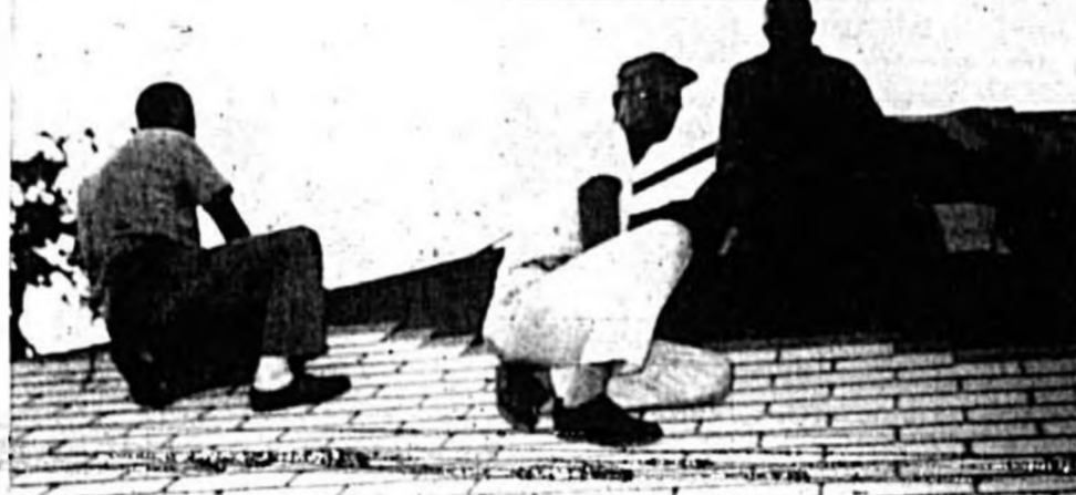
WORKMEN took advantage of the recent school holidays to begin improvements at the Geneva School starting with a new roof expected to be completed this week. (Herald Photo)
