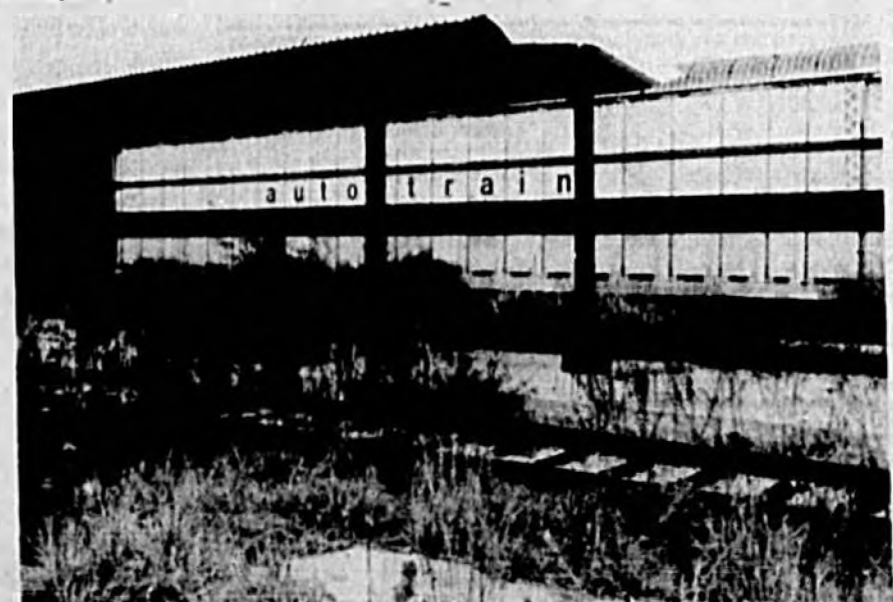
Sanford's Auto-Train terminal looks like a graveyard as final action is awaited that could turn the once-busy facility into a major train depot again.
