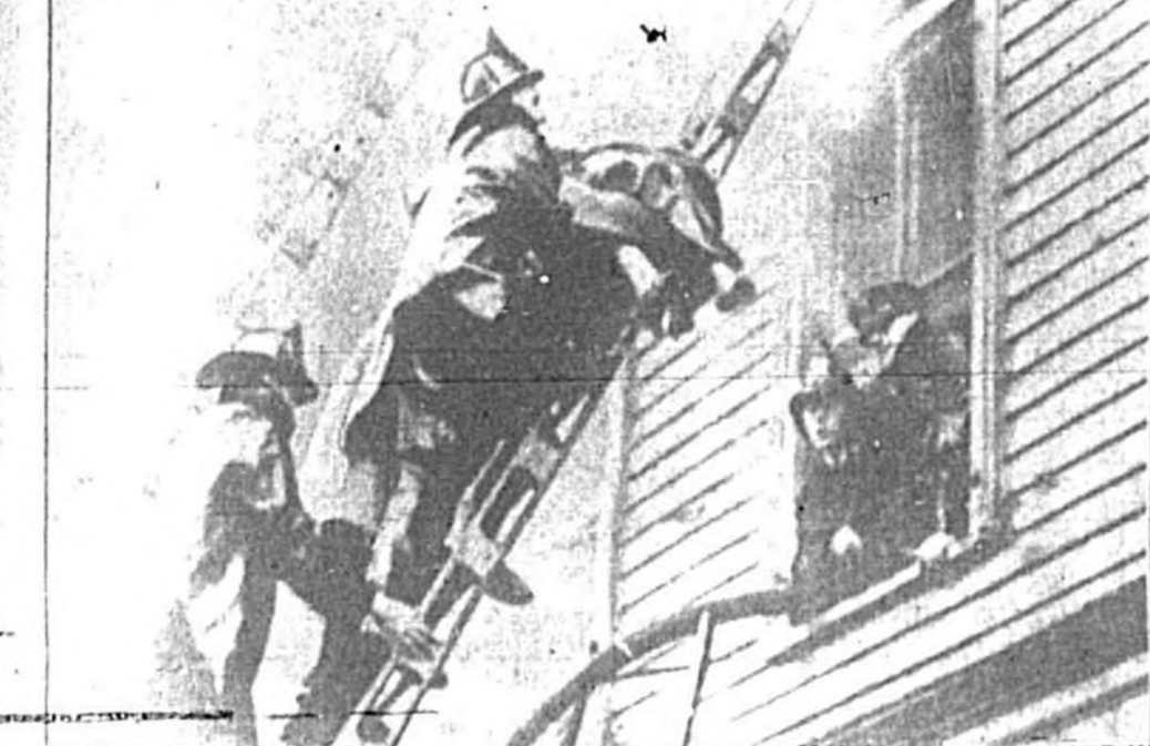
Five children were killed and five others injured in a fire which started at a play in a school building in Lawrence, Mo. The fire broke out at 10:30 a. m. and was extinguished by 11:30 a. m. The cause of the fire was determined to be a match thrown by one of the children.
