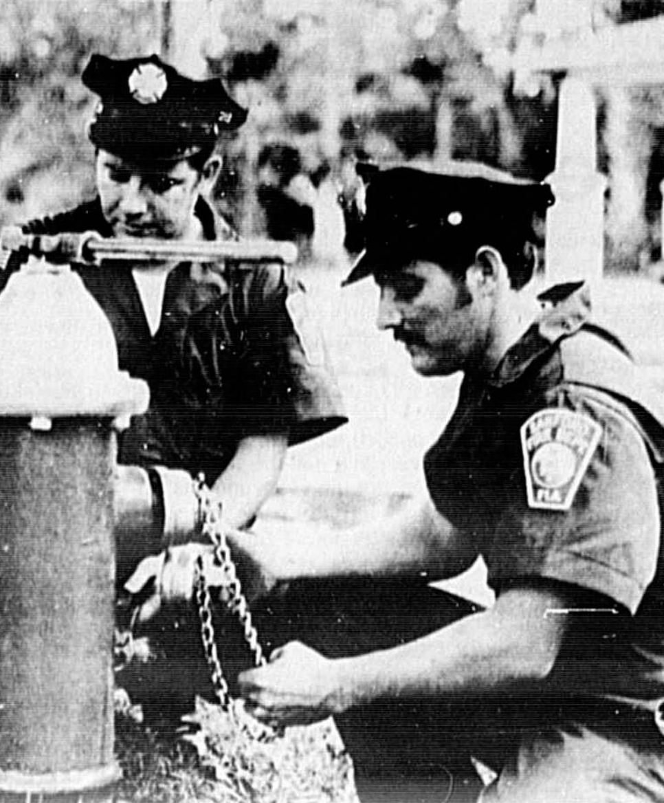
SANFORD FIREMEN began annual check Thursday of over 400 fire hydrants in the city. Above, Randy Mawby, left, and Herman Brown inspect and test a hydrant. Fire Chief G. M. Harriett said all of the 40 hydrants checked Thursday were found to be operational.
