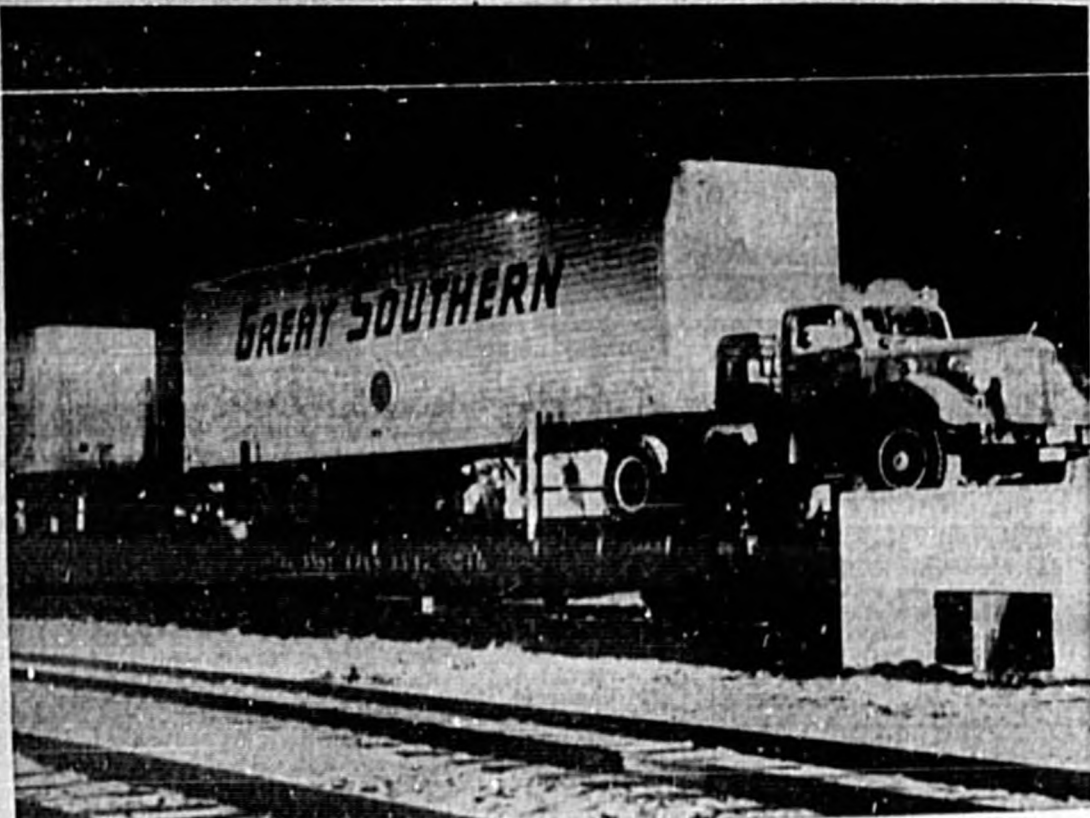
THE SOUTHEAST'S FIRST trailer-truck piggy-back train combination rolled into Miami from Jacksonville this week, the event inaugurating a regular service by Great Southern Trucking Company between the two cities. The flat cars provided by the Florida East Coast Railway to accommodate the huge trailers are fifty-five feet long and were specially designed as were the ramps and trackage at each terminal to insure the speedy loading and unloading of the trailers. Great Southern, a division of Ryder System, Inc.—the country's largest exclusive truck rental concern—is the largest common carrier in the Southeast. As the trailers move off the train they are sped immediately to their final destination.
