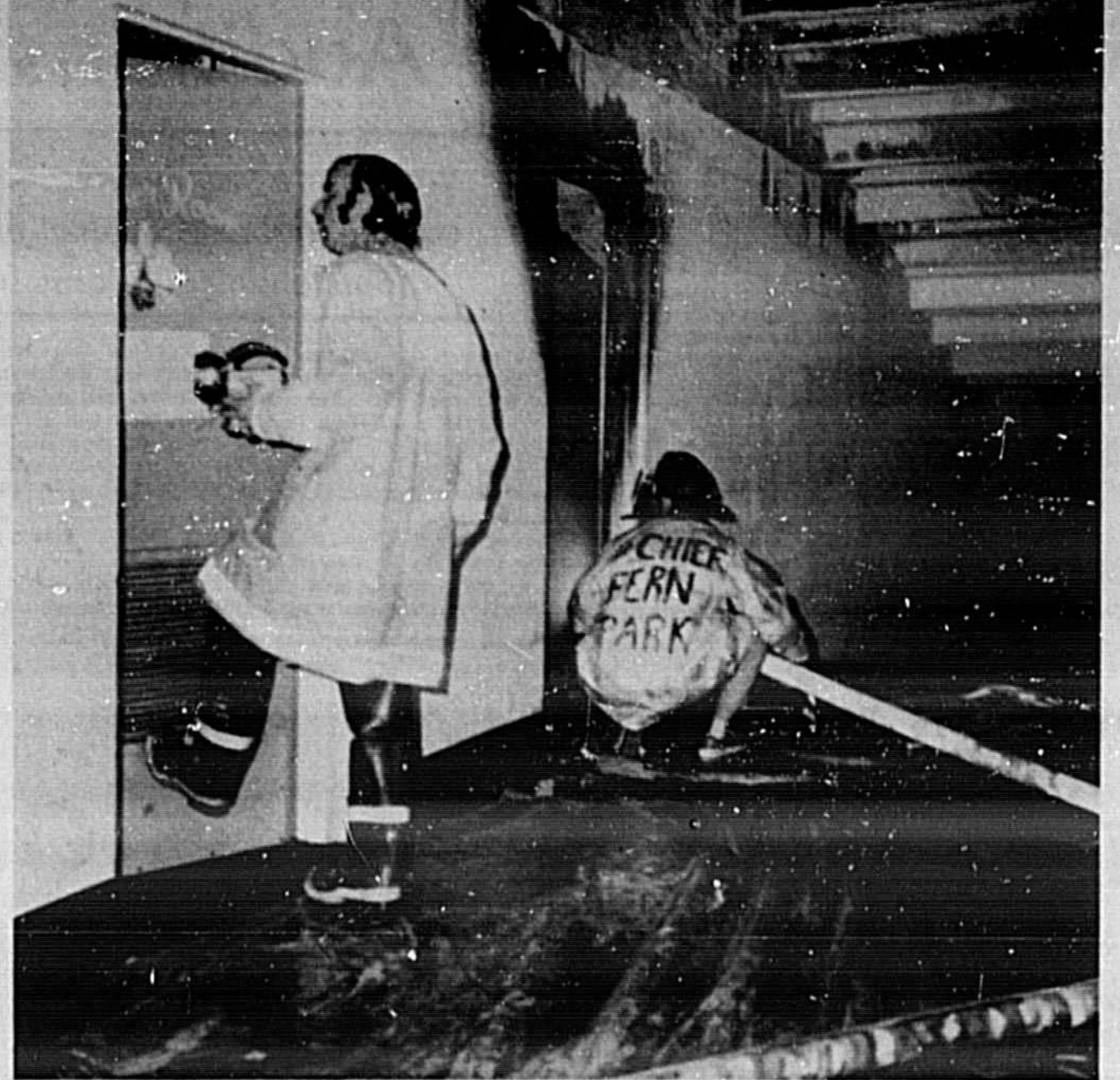
FLAMES were contained in the fireproof Jai Alai Fronton at Fern Park this morning but smoke caused considerable damage to the plant, according to Gordon Hulbert, general manager. The blaze was contained in the tele-wager girls' room, being sprayed in this photo by firemen as another enters a powder room. (Bill Vincent Photo)
