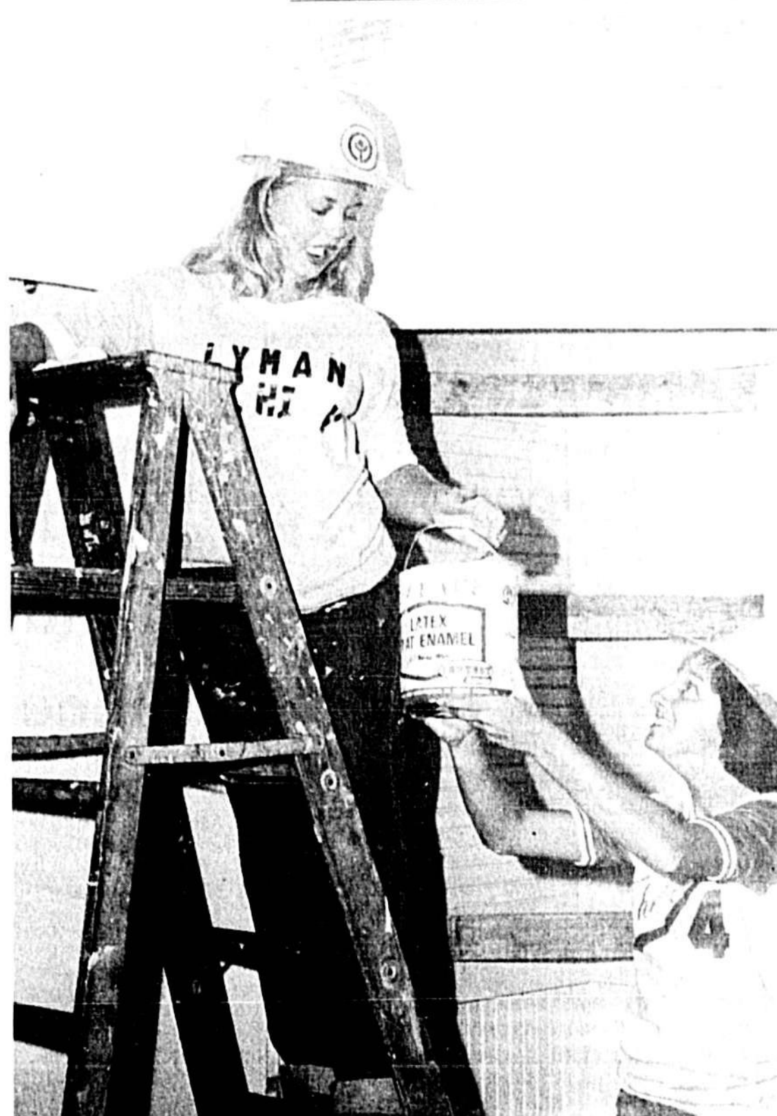
Jenny Scarbrough (on ladder) and Renee DiCarlo put finishing touches on paint job at Nature Center building.
