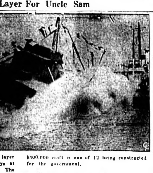
The YF 286, a combination mine layer and freight lighter, is launched sideways at the Sullivan Drydock, Brooklyn, N. Y. The $300,000 craft is one of 12 being constructed for the government.
