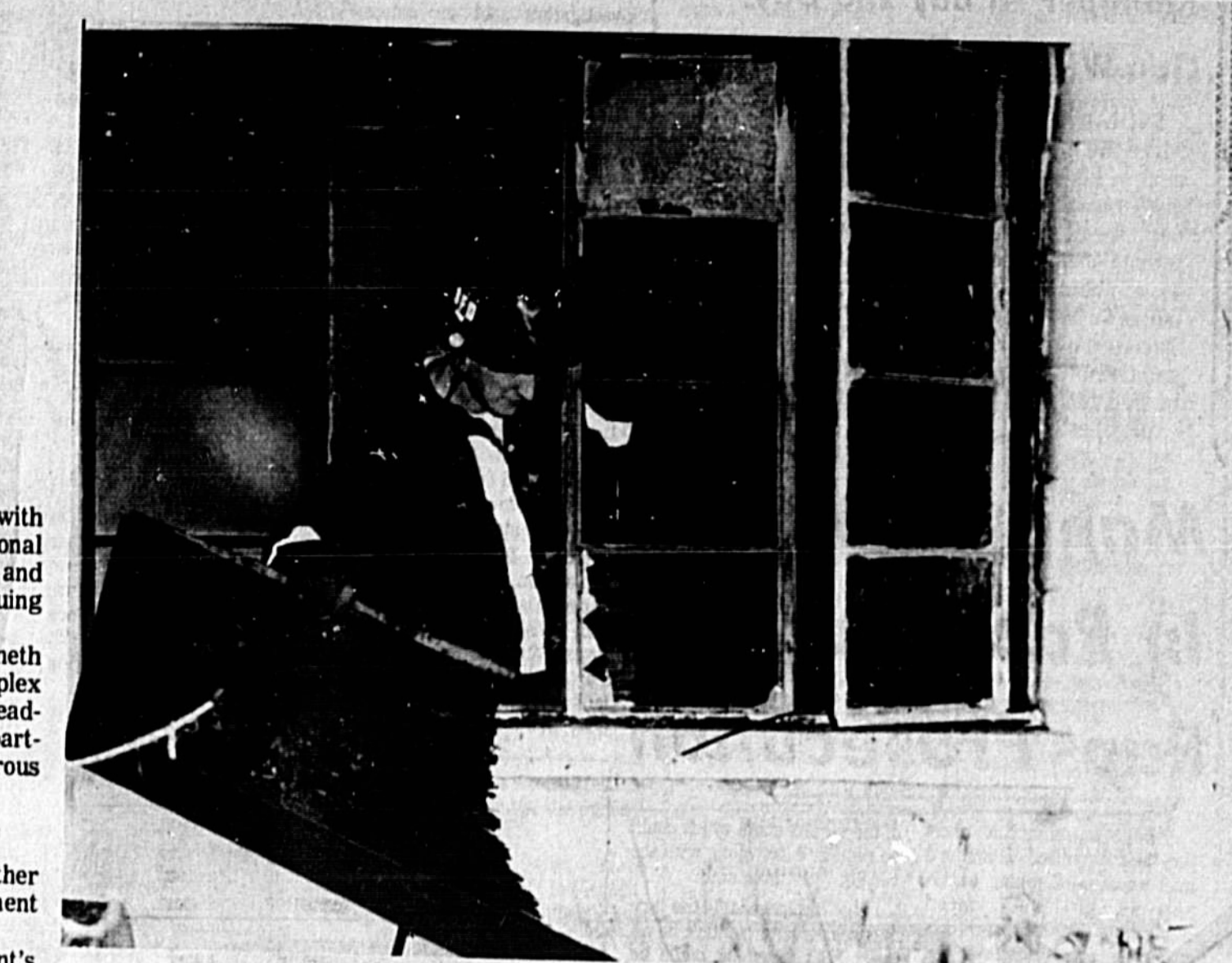
FIRE DAMAGES SANFORD HOME Sanford Fireman Bill Price removes burned material from Jerry Walker residence at 516 E. Fifth Street after blaze which occurred Tuesday. One person reportedly was slightly injured in the blaze. Cause of the fire was not immediately determined. Another fire, in Midway, resulted in a fatality Tuesday night. Details in Action Reports, Page 2-A.
