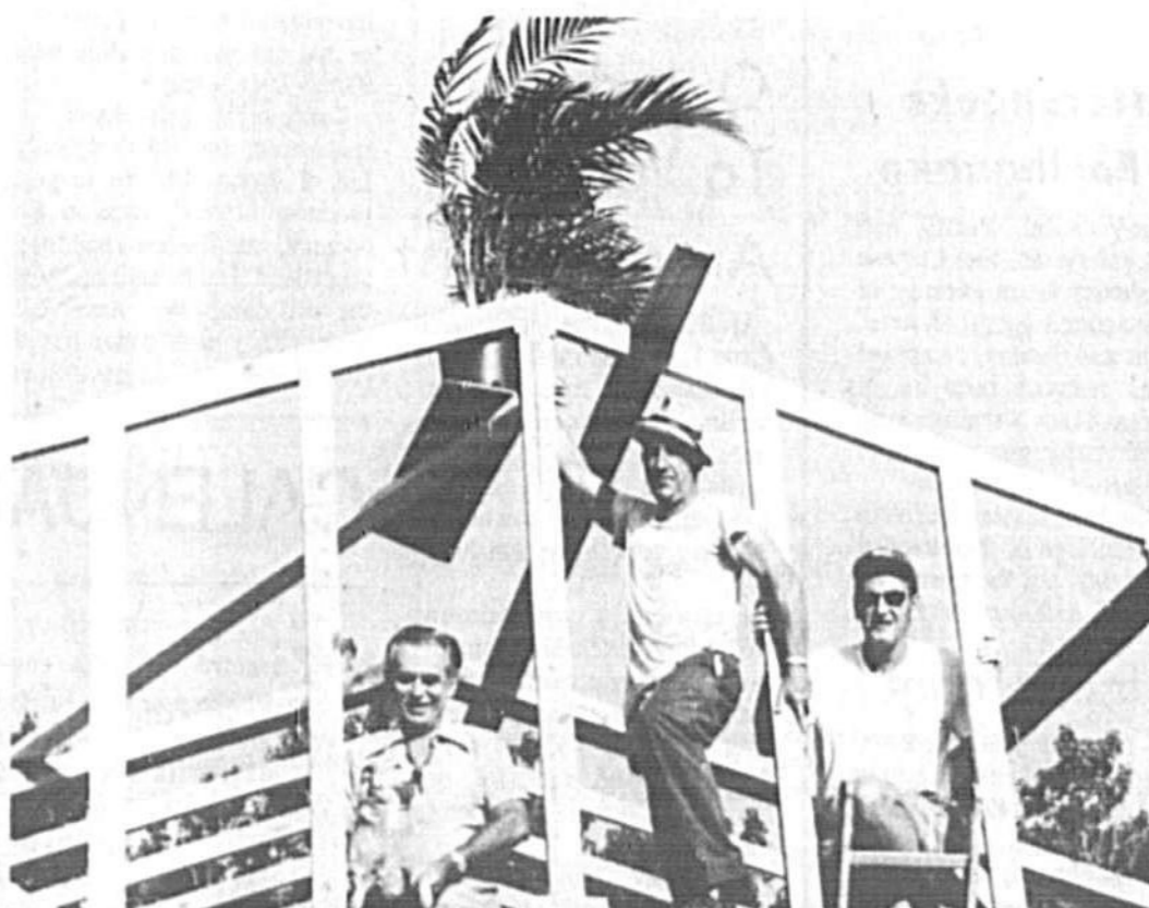
Volunteer workers John Matthews (left) and John Girtler flank Building Chairman John Fehr at a tree-topping ceremony this morning at the B. Duke Moody Branch 147 Fleet Reserve Assn. building on SR-46, west of Sanford. The building is getting a $30,000 meeting hall addition. (Herald Photo by Bill Vincent Jr.)
