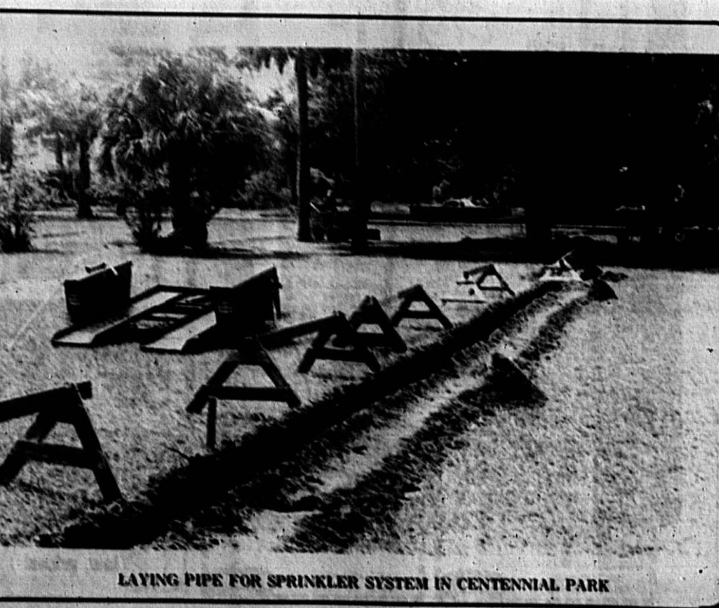
LAYING PIPE FOR SPRINKLER SYSTEM IN CENTENNIAL PARK
