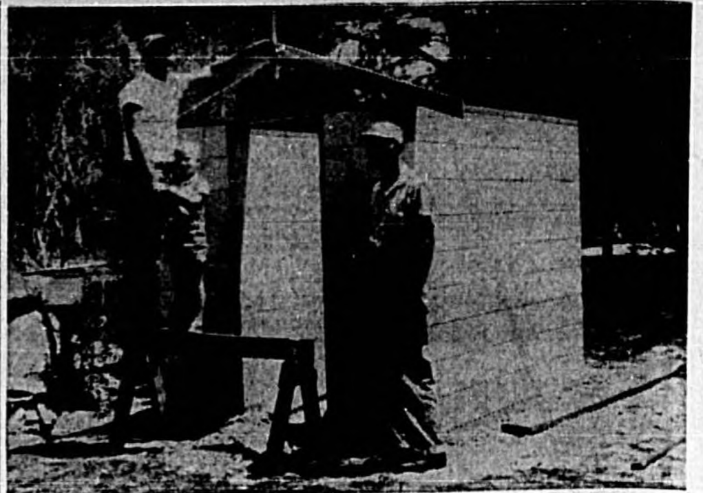
A NEW PUMP HOUSE is under construction at the Enterprise Cemetery and when electricity and the pump are installed, another dream will come true for the community. In the past, all water has come from a centrally located hand pump. A pipe line running the cemetery's full length will be laid and 12 faucets and hose connections will be installed. Shown working on the building is Wilbur Bruce, president of the Cemetery Assn., son, Joe and Sidney Emanuel, association trustees. (Cox Photo)
