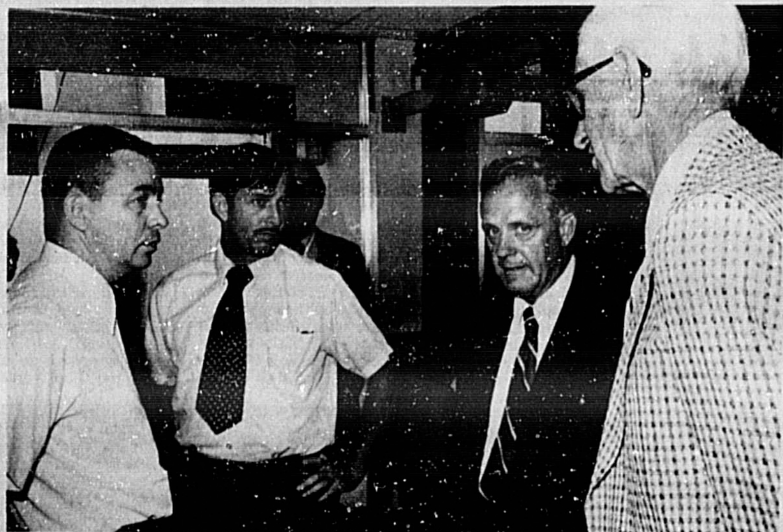
Circuit Court Judge Robert B. McGregor, second from right, discusses fire situation with Assistant State Atty. Bill Staley, left, County Court Judge Wallace Hall and Sheriff's Capt. J. Q. "Slim" Galloway, right, before inspecting fire-damaged county jail.
