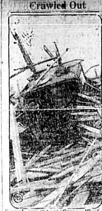
George Warfel, an chauffeur of Miss Pickford, crawled out from under the roof of the limousine, a dance hall, came hurling through the air and onto his car during a wind storm.
