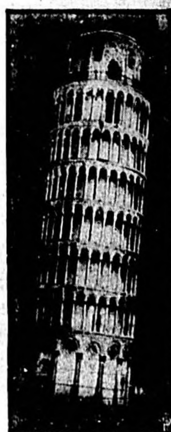
THE LEANING TOWER of Pisa, expected to fall within 50 years unless something definite is done soon, may be taken apart stone by stone and rebuilt, according to a plan suggested by Prof. Giovanni Doga of the University of Rome. The tower would be re-assembled on a massive concrete foundation guaranteeing the landmark's life for another 750 years. At present, the topmost point is 17.15 feet out of plumb, with the tilt increasing at the rate of about .027 inches yearly.
