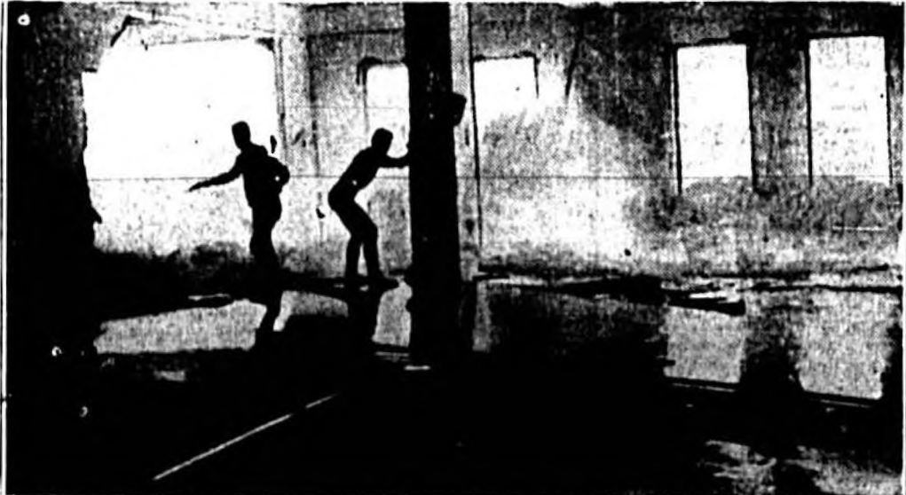
Miami's million dollar pier was damaged heavily when the hurricane lashed southern Florida, killing seven persons, and causing property damages estimated at $2,000,000. A short time after these daring youths quit playing in the interior of the dance hall as it was swept by gigantic waves, the flooring and walls were washed to sea. (Associated Press Photo)
