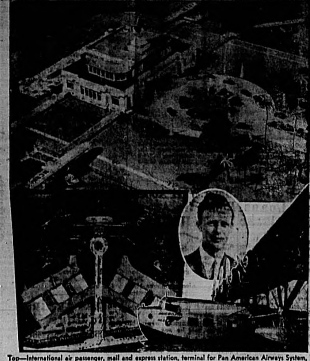
Top—International air passenger, mail and express station, terminal for Pan American Airways System, now under construction in Miami at the world's largest commercial marine aviation base.
