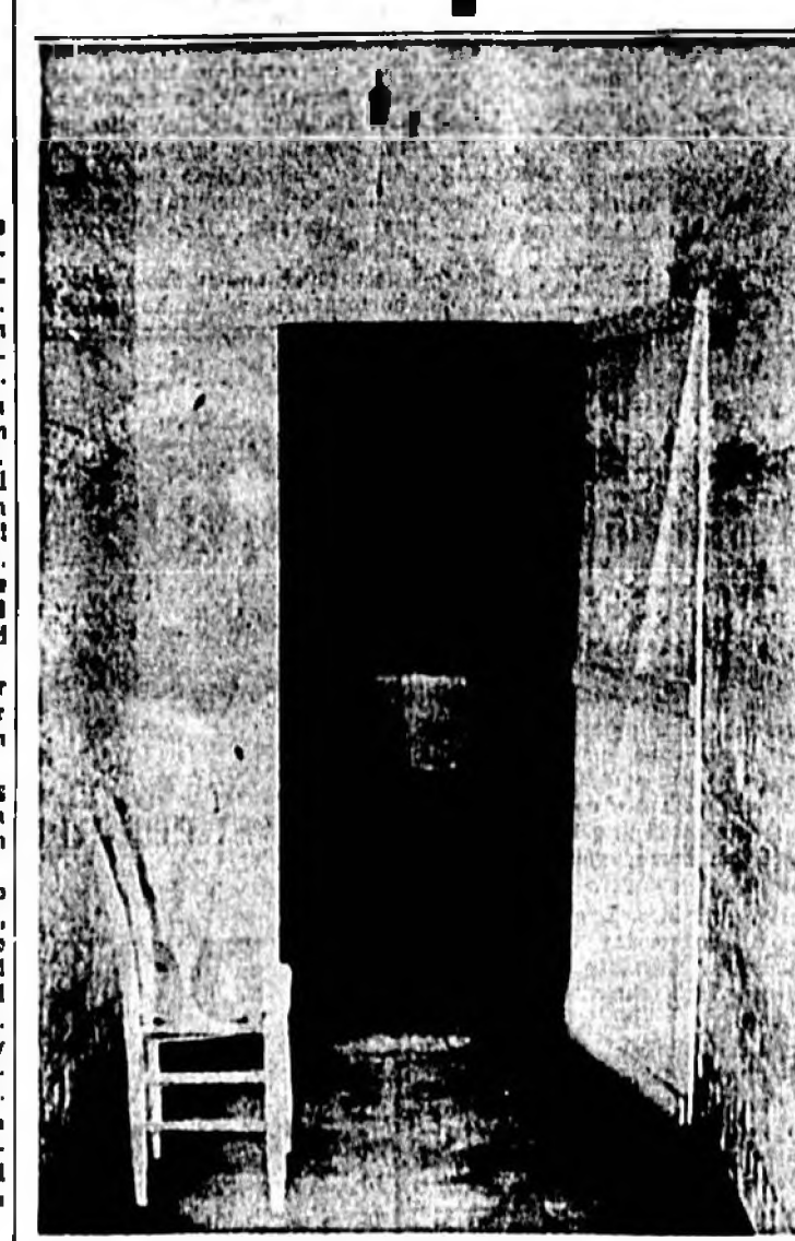
ENTRANCE TO FORMER BULL PEN now being used for general office of the Seminole County Health Department. Note the old-fashioned drop light, the makeshift door and the dungeon-like appearance of the interior. Building was former jail. (Photo by Bergstrom)
