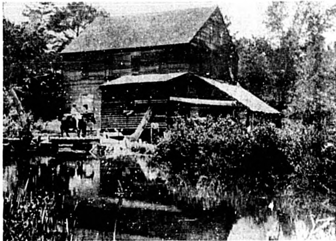
The original Felbeck mill (right) which was built by slaves in 1828 near Columbus, Ga. Its framing and wood weatherboarding were hand dressed lumber and joined together with wooden pegs. The mill continued to stand until 1944 when the federal government acquired the site and demolished it.
