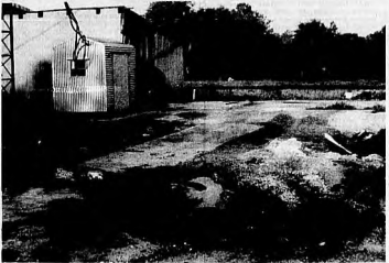
Old Chemical and Fertilizer plant subject of condemnation action.
