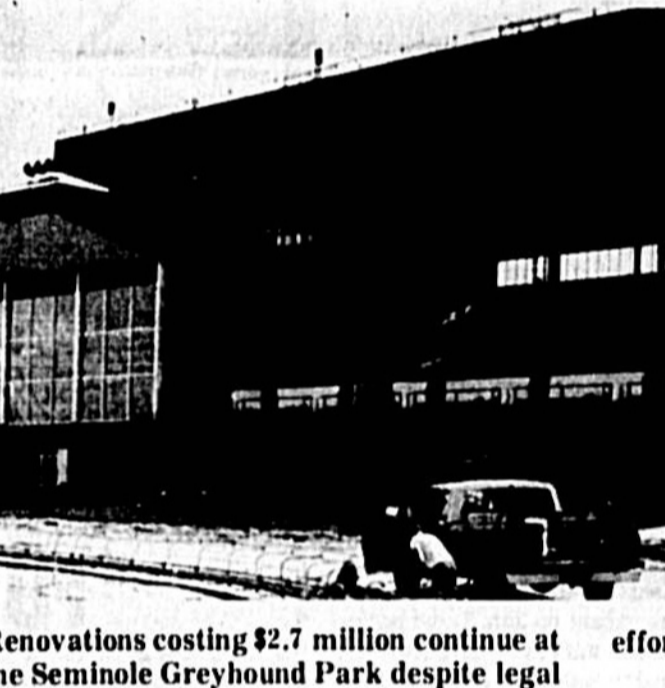
Renovations costing $2.7 million continue at the Seminole Greyhound Park despite legal efforts to stop the grand opening.
