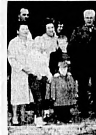
GROUND-BREAKING for the new First National Bank of Delbarton, to be located on Highway 17-92 between Seminole and Catalina Drives, was conducted Friday. Pictured with the group directors and board members present for the occasion are Albert J. Govan, chairman of the
