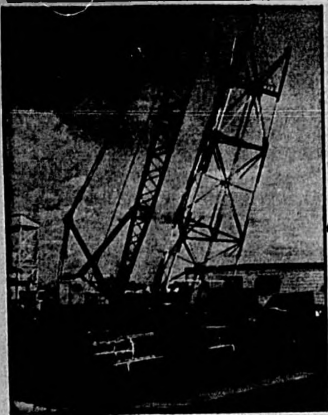
WORKMEN at Sanford Naval Air Station, with the help of a 100-foot crane, hoist a new radar weather-tracking tower into position. In foreground is access ladder which was mounted along side of the tower. (Navy Photo)
