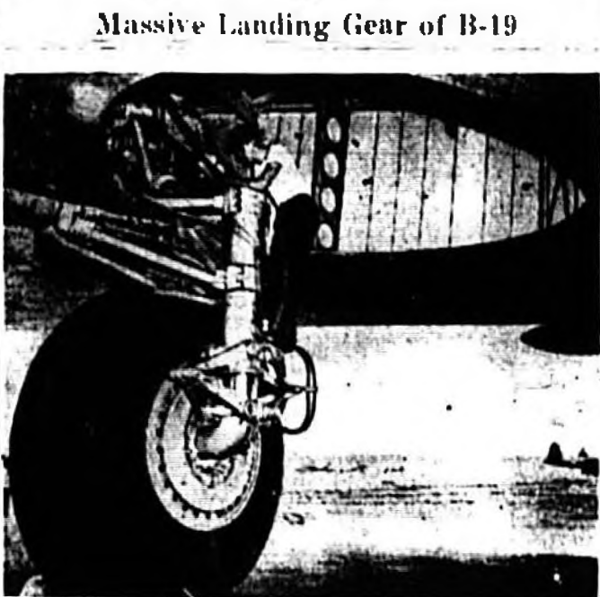
Massive Landing Gear of B-19
