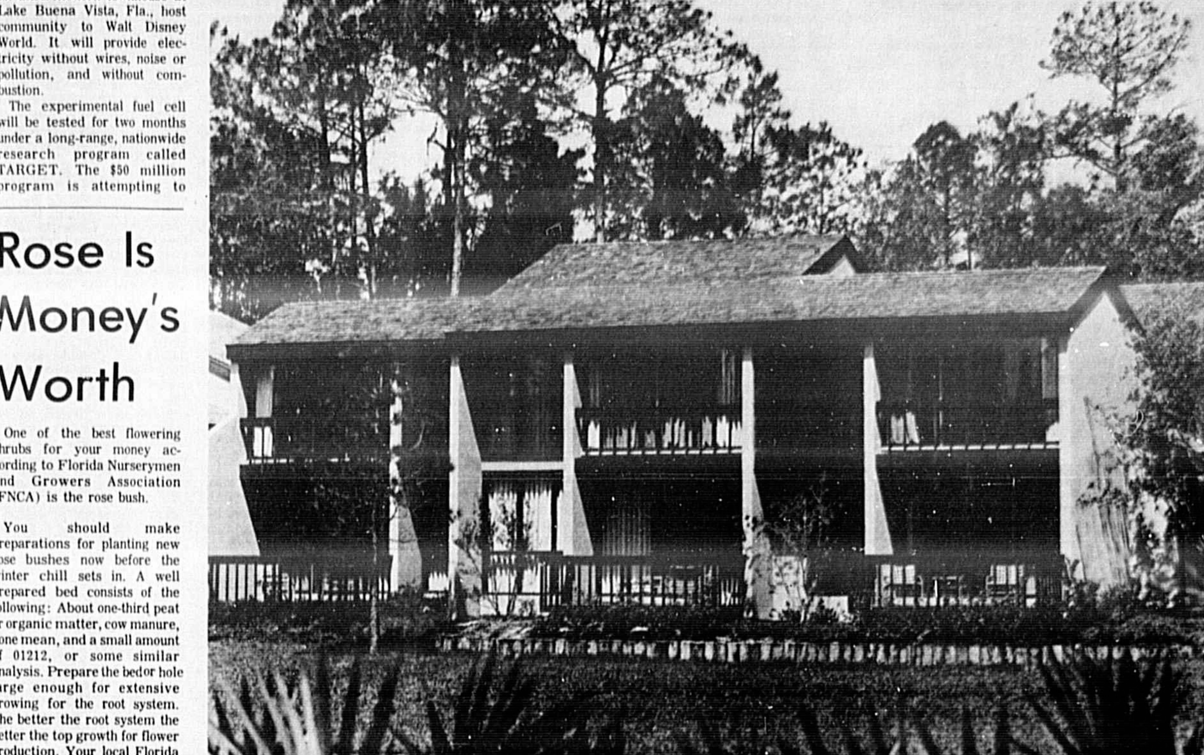
ELECTRICITY for one of the units in this townhouse complex at Lake Buena Vista, host community to Walt Disney World, will be produced by a natural gas fuel cell. The fuel cell powerplant, installed by Florida Gas Company, produces electricity on site and without combustion. The only by-products are water vapor and harmless carbon dioxide.
