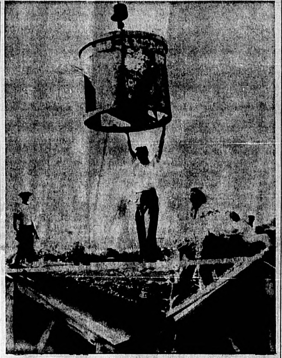
A WORKMAN swings aloft as the crane operator raised the concrete bucket a little too high. Crews began to pour the roof of First Federal's new bank on First Street this morning. (Herald Photo)
