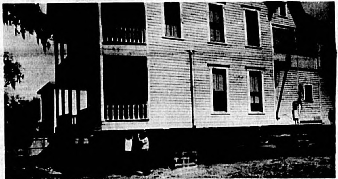
The Bowlin's historic home rests on six-foot wooden blocks that resemble orange crates.
