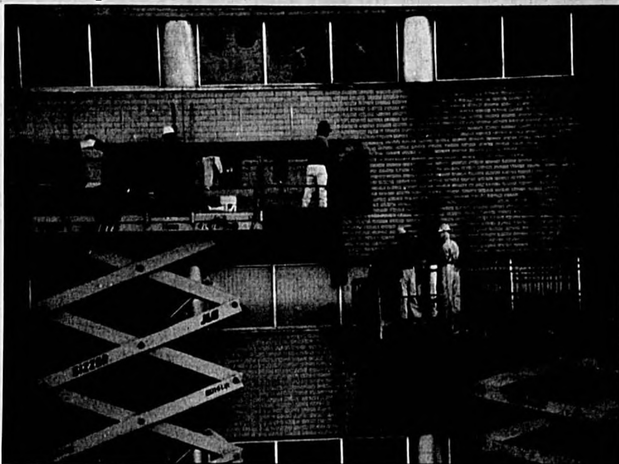
Workers are continuing their work on correcting a mold problem at the Seminole County Public Safety Building on Bush Boulevard using a SIZZOR lift to reach the second and third floors.
