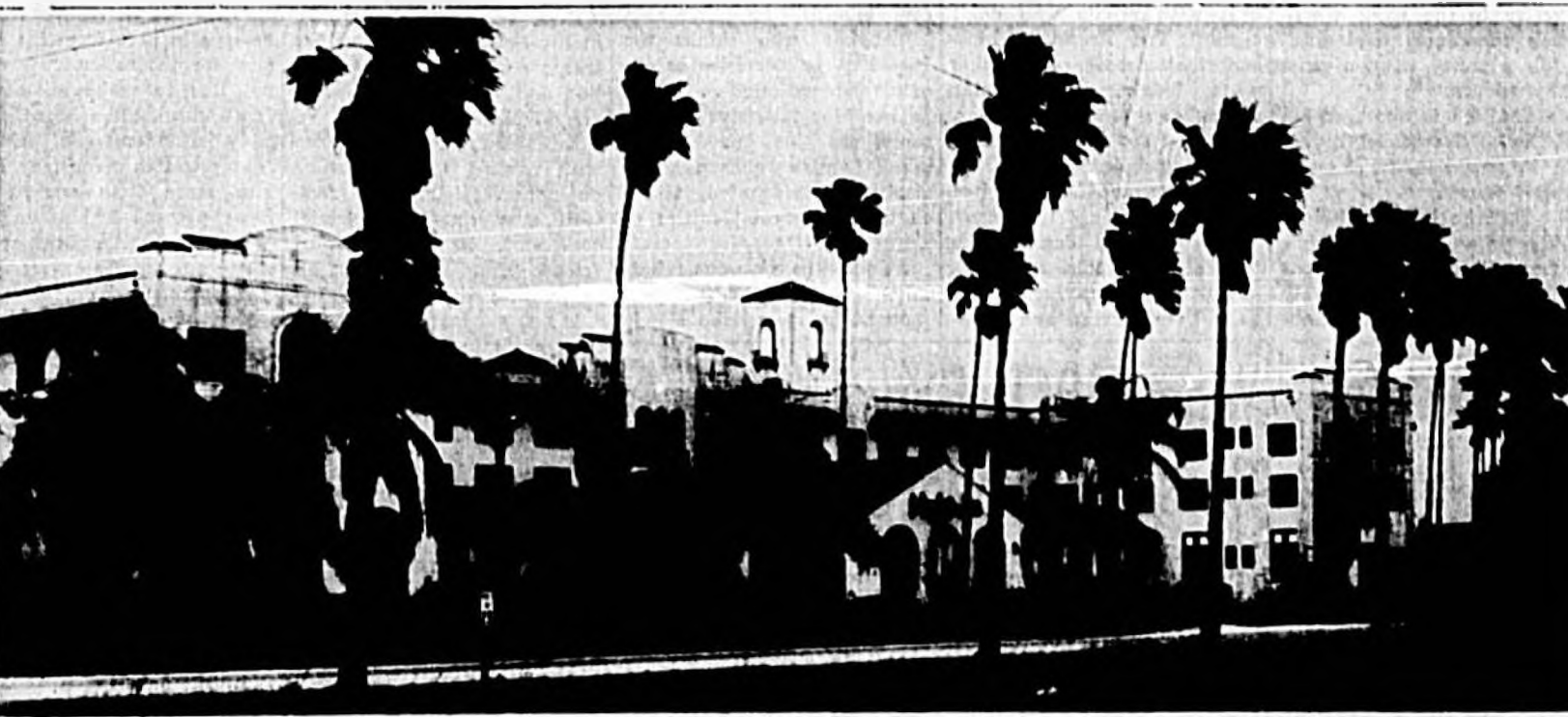
CITY OF SANFORD and county will lose $25,000 annually in taxes when the Mayfair Inn (above) and its annex (motel) are taken over in about six weeks as dormitory and classrooms by the Sanford Naval Academy, to be known as "Commandore Barry Hall." Official announcement of the transaction is to be released in New York City Wednesday by J. P. Wieggers, president of the Bernarr Macfadden Foundation, a non-profit organization, sponsors of the academy, and Horace Stoneham, president of the National Exhibition Company (San Francisco Giants). (Herald Photo)
