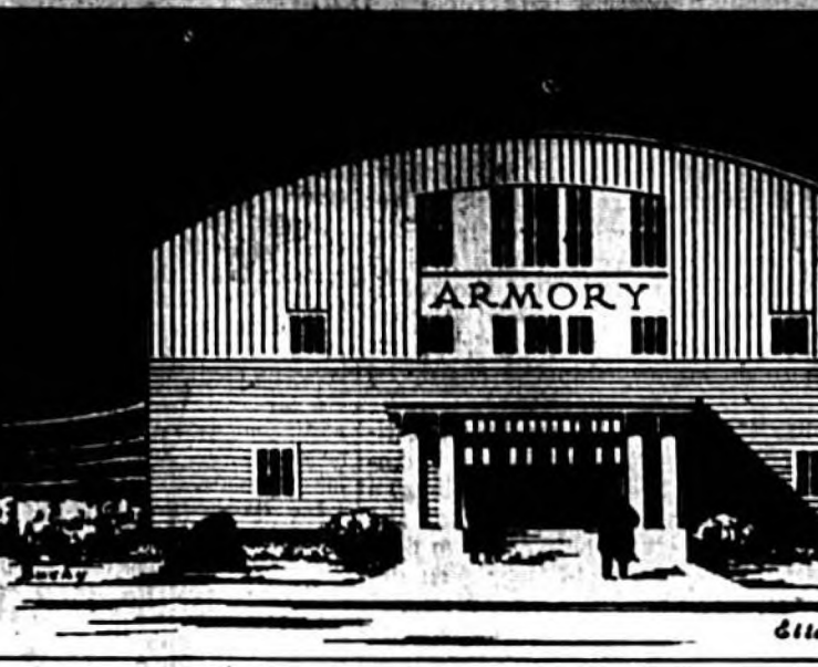
Architect's drawing of the Seminole County Armory now under construction on property donated by the City of Sanford, located on East First Street. When completed, the upper floor of the building will afford the largest auditorium in the city. The WPA granted $24,000.00 to this project, and an additional $5100.00 has been contributed by the City of Sanford, Seminole County Commissioners and the State Armory Board.
