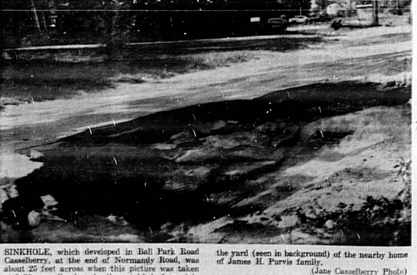
SINKHOLE, which developed in Ball Park Road Caselberry, at the end of Normandy Road, was about 25 feet across when this picture was taken at 9:30 a.m., Sunday. Another sinkhole formed in the yard (seen in background) of the nearby home of James H. Purvis family. (Jane Caselberry Photo)
